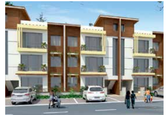
TDI Casa Floors, Mohali
